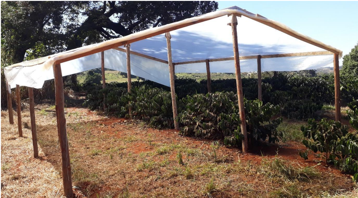
Fig. S1 Design of rainfall exclusion treatment in field experiment II. Rainfall exclusion was achieved through the installation of translucent nylon (polypropylene) fixed on twelve 3.2 m high eucalyptus wood logs, buried 0.60 m deep in the soil with three wood logs 3 m distant from each other. Every eucalyptus wood log was arranged on each posterior side and in the middle of the coffee line. A translucent nylon piece of 0,2 micrometers was fixed on top of wood logs using a wooden piece of 5x7 cm with a small hobnail, covering a total of 81 m 2 of rain exclusion area.
