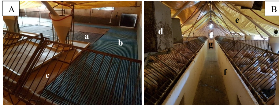
Figure 6 - A and B - Nursery stall floor: a) metal mesh floor in the central area, b) polyethylene mesh material around the stall, and c) concrete floor in two specific areas to support the feeders. d) Heat exchanger, near the corridor door; e) yellow canvas, covering the stalls to maximize the heating; f) walls at the corridor, dividing the room in two areas; g) door.
